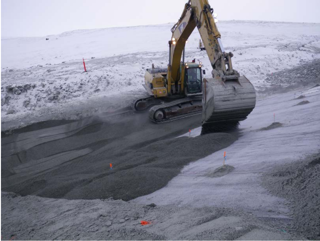
Photo 6: North Dam – Excavator placing overliner material on slope.
