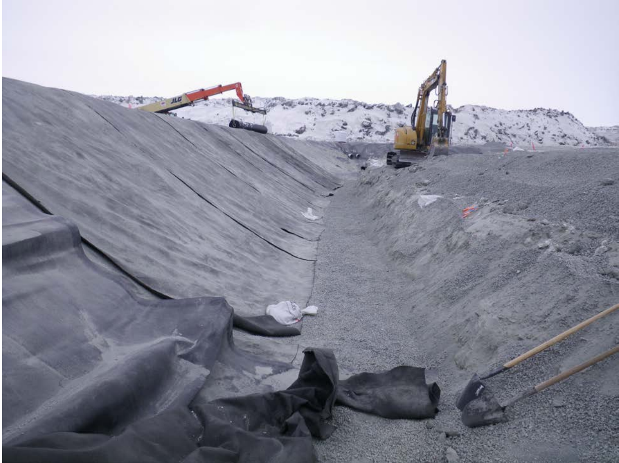
Photo 4: Diversion Berm – View of replaced HDPE liner at approximately station 050 looking west towards the culverts through the Primary Road.
