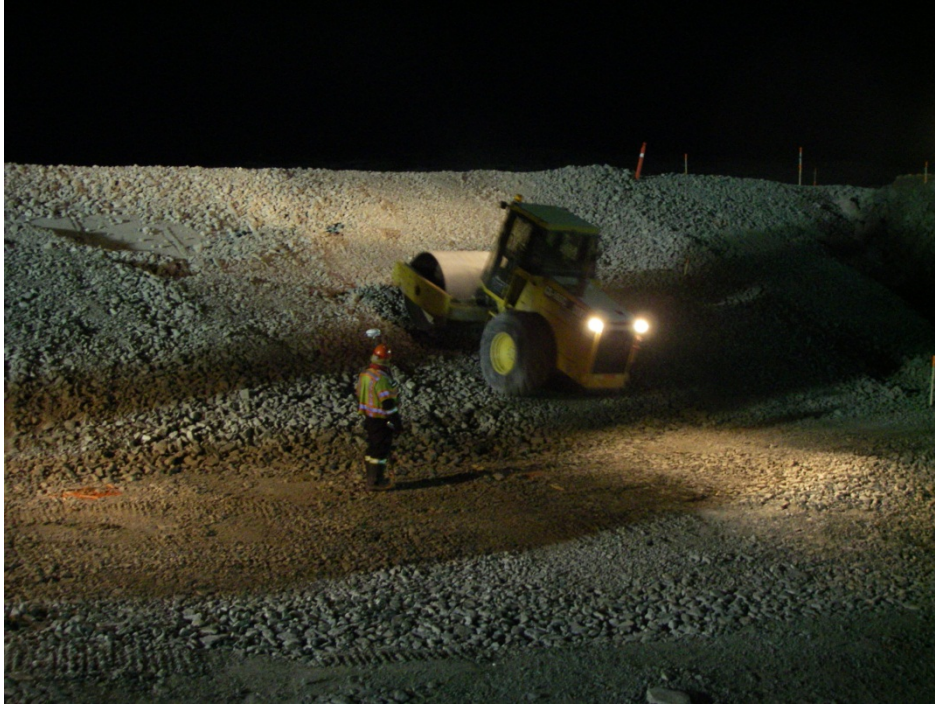
Photo 9: North Dam – compacting the second lift of transition material. Photo looking north-west from Sta. 0+60.
