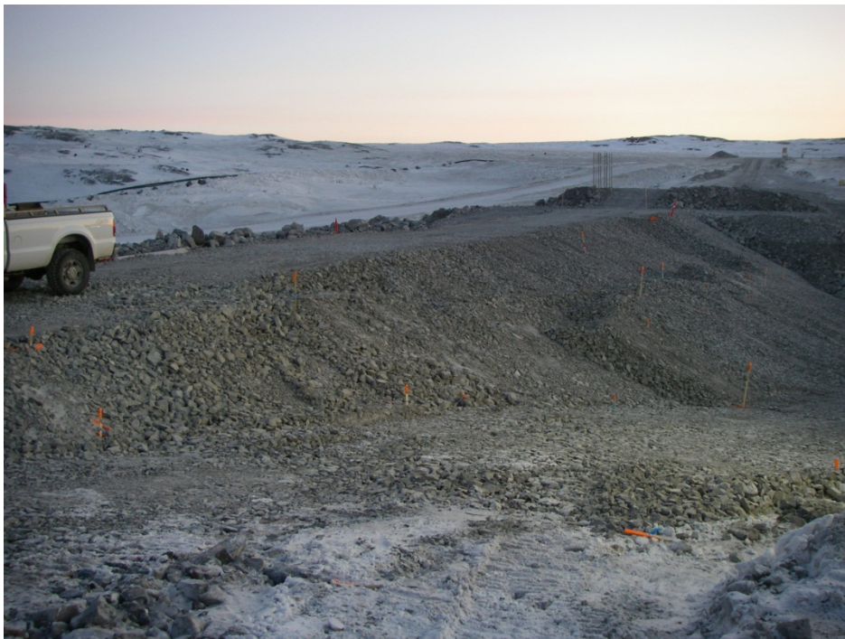
Photo 12: North Dam – completed transition on the crest of the dam. Photo looking north from Sta. 0+20.
