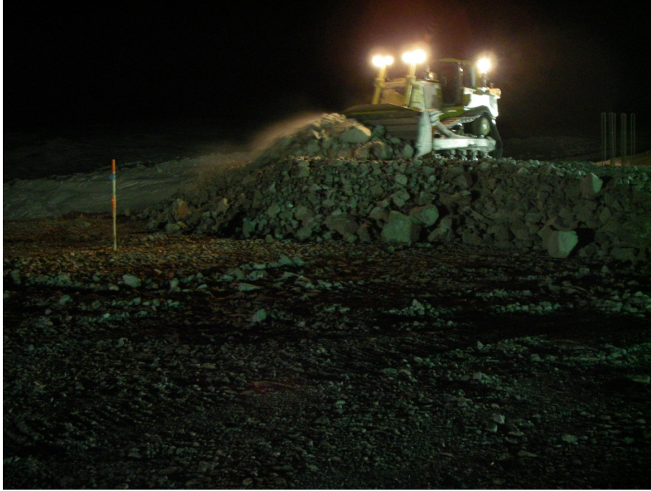
Photo 11: North Dam – progress photo of the final lift of ROQ. Photo looking north-west from Sta. 1+00.
