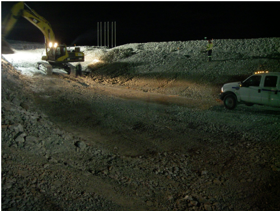
Photo 10: North Dam – finished transition material blanket up to elevation 32.5. Note the windrows perpendicular to the slope, indicating that further compaction is required. Photo looking west from Sta. 0+85.
