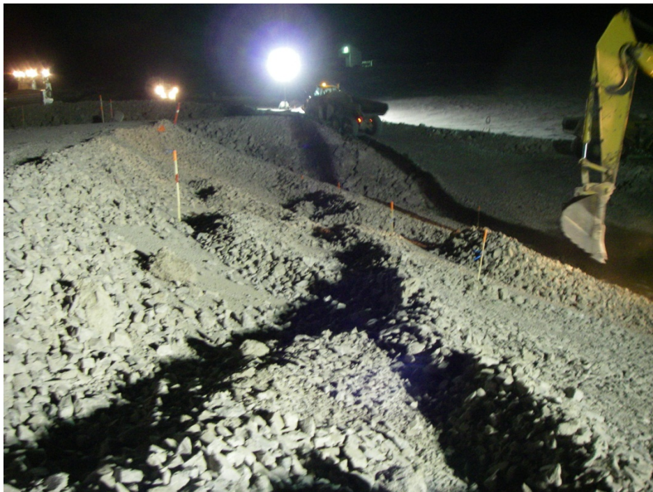
Photo 7: North Dam – Progress photo of transition material placement. The three consecutive lifts are clearly visible. Photo looking north-east from Sta. 0+50.
