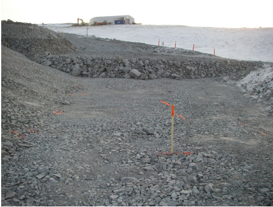
Photo 13: North Dam – progress photo of the first lift of ROQ at the toe of the core. The stake in the foreground is marking the extent of the area approved for covering with ROQ. Photo looking north-east from Sta. 0+55.
